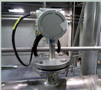
In year 2019 more units was purchased for the old  $H_2SO_4$  plant to replace conductive analyzers. One at the outlet of plant to storage tanks, second one for feed line to drying tower and third one for return line of the final absorption tower.
