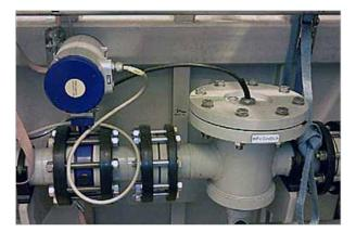
Installed sonic velocity and conductivity sensor
