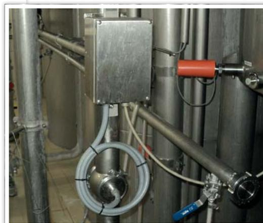
**LiquiSonic sensors are positioned in main pipings or vessels**
